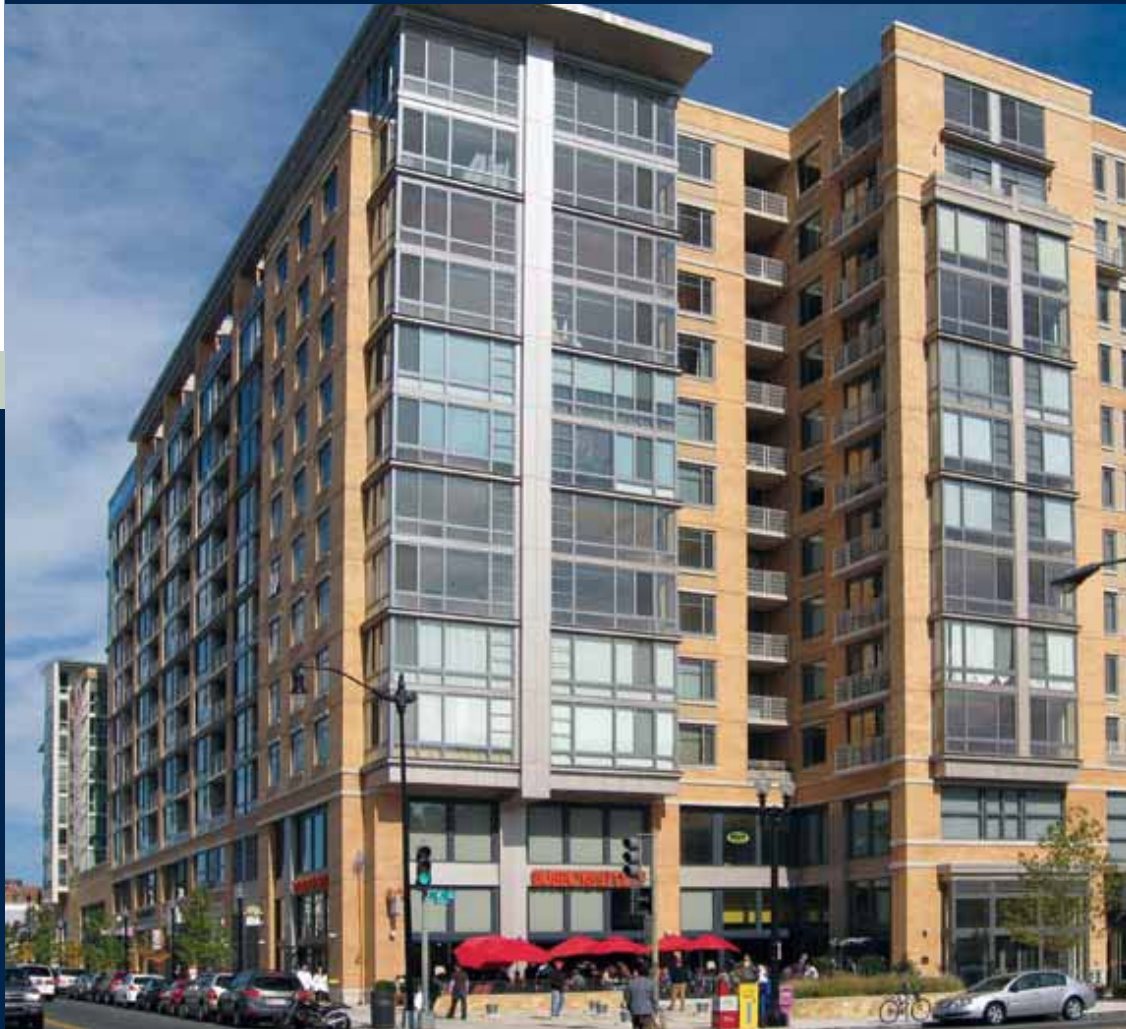
CityVista delivered 685 residential units, 117,000 sq. ft. of retail space, including a 55,000 sq. ft. urban lifestyle Safeway grocery store in 2007–2008
